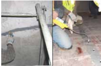
USA- San Francisco, CA Honda car dealer structural floor repair ETI and pasteover above and below crack surface
