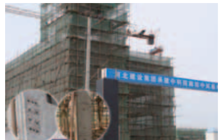
China- Hebei Steel structure anchoring
