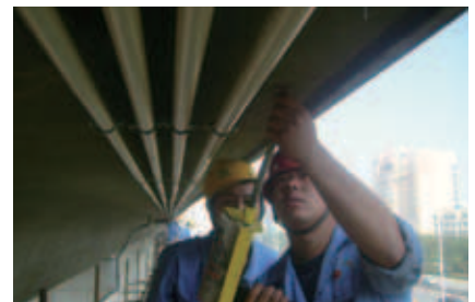
China- Tianjin Light rail anchoring
