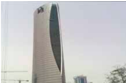
Qatar- Doha Navigation Tower Dowelling of floors to core wall
