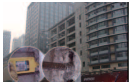
China- Beijing Albemarle Building Renovation work
