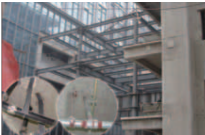
China- Beijing Steel structure anchoring
