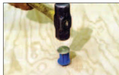
Wood-Form Insert Installation Sequence
