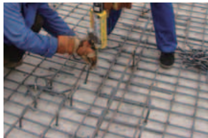
China- Beijing Wintertime bridge repair
