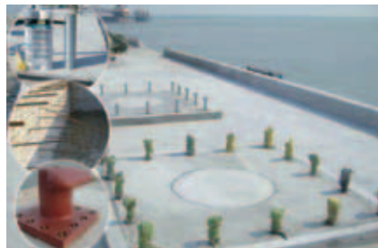
China- Shandong Seaport Loading arm, equipment anchoring
