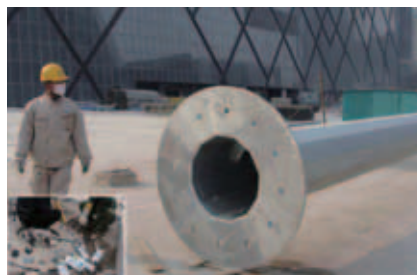
China- Beijing CCTV Building Used in steel anchoring
