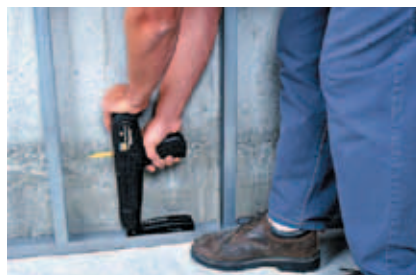
UAE- Dubai Dubai Mall P.A.T. system used for interior finishing work
