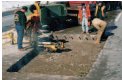
USA- Illinois Wintertime highway repair
