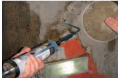
China- Beijing Damp condition leak repair
