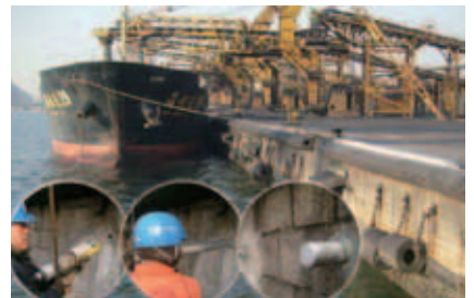
China- Henan Seaport Fender, mooring, railing large diameter anchoring
