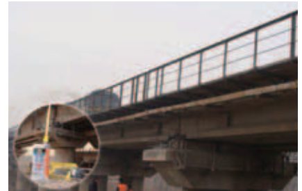
China- Shandong Railway bridge renovation
