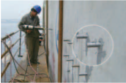
China- Hebei Qinhuangdao Caisson tube anchoring
