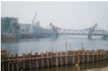
China- Tianjin Seaport Damp condition fender anchoring
