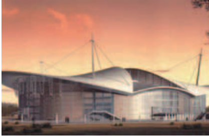
China- Beijing Olympic Velodrome Stadium Roof structure anchoring
