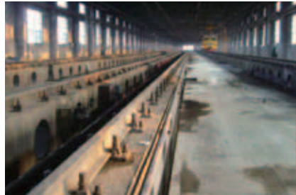
China- Harbin High speed railway anchoring
