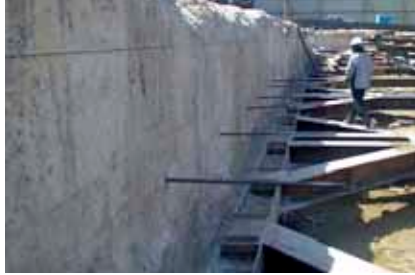
Thailand- Hua Hin Intercontinental Hotel Wet hole rebar installation
