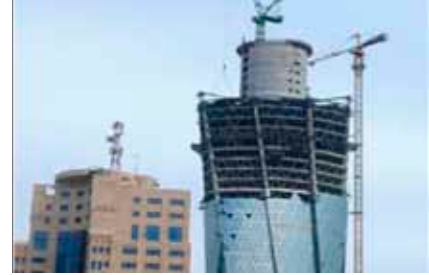
Qatar- Doha Doha Tower Dowelling of floors to core wall
