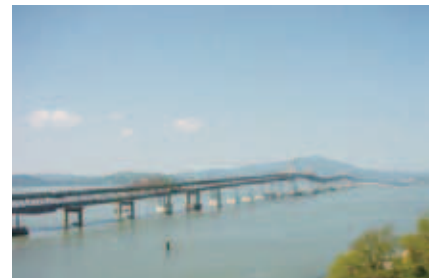
USA- California Richmond-San Rafael Bridge Seismic upgrade
