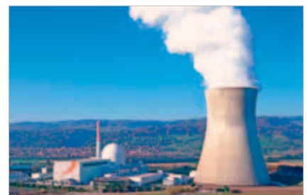
Germany Used in nuclear power plant
