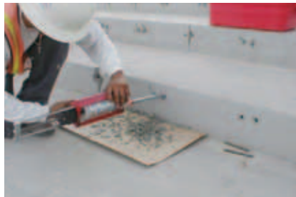
USA- Wisconsin University of Wisconsin Stadium seating installation
