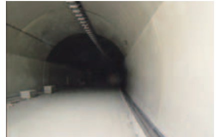
Slovenia Used in fixture installation in tunnel
