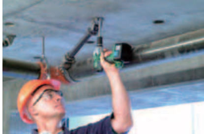
USA- California Pipe system anchoring
