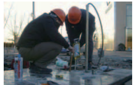
China- Tianjin Steel structure anchoring
