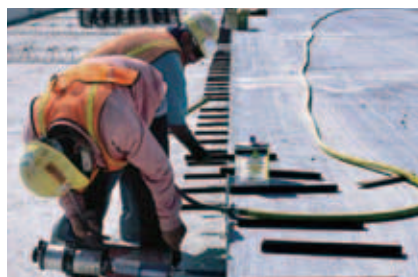
USA- Texas Ellington Airfield Airport runway extension
