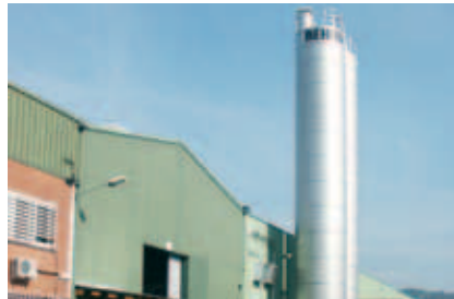
Germany- Troisdorf Used in silo anchoring
