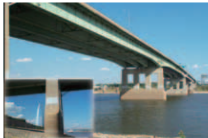
USA- Missouri Poplar Street Bridge Seismic upgrade
