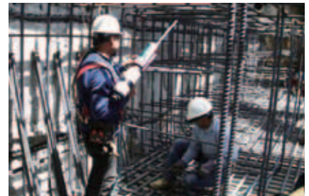
USA- California San Francisco-Oakland Bay Bridge Seismic upgrade
