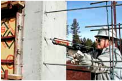
California- San Diego AT-HP® Used in dowelling for column enlargement
