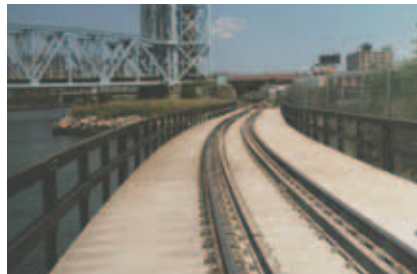
USA- New York Oak Pointe Railroad Bridge Bridge and track renovation
