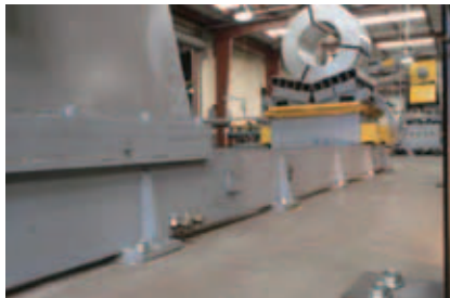
USA- California Factory machinery anchoring
