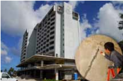
Pacific Islands- Guam Charter House Structural crack repair
