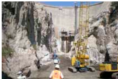
USA- California Tujung Dam Seismic Upgrade
