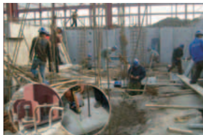
China- Tianjin Steel anchoring
