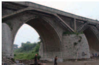
China- Henan Seismic upgrade of bridge
