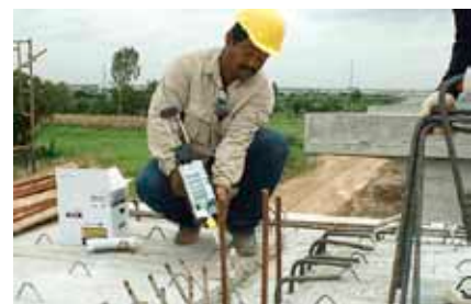
Thailand- Bangkok IRR Elevated Highway Rebar dowelling
