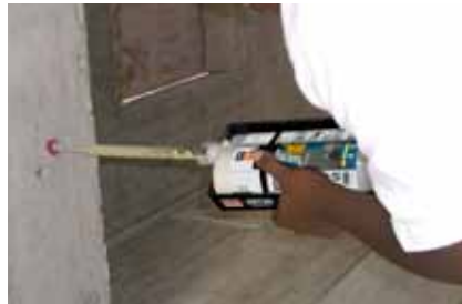
China- Beijing Fixture anchoring in hollow block wall with screen tube system
