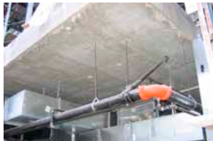
U.S.A.- New York City parking garage Drop Ins used in interior mechanical work
