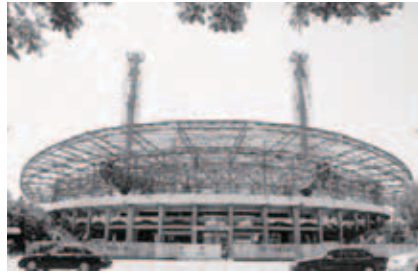
China- Beijing Worker's Olympic Stadium Renovation work
