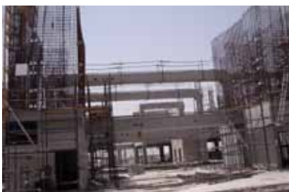
UAE- Abu Dhabi ET-HP™ used in Yas Island Ferrari Building at Abu Dhabi F1 race track
