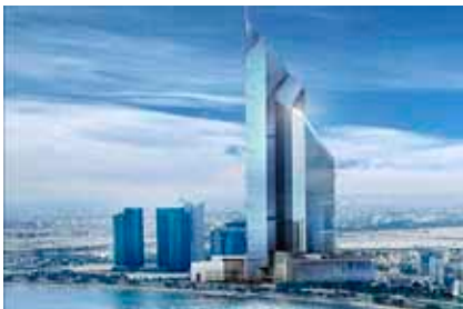
Qatar- Doha Dubai Tower Dowelling of floors to core wall
