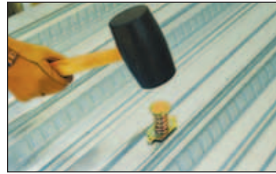
Metal-Deck Insert Installation Sequence
