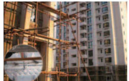
China- Tianjin Winter time and wet weather anchoring
