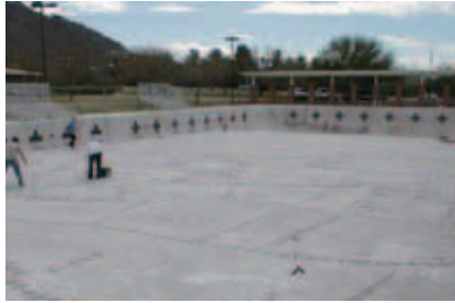
USA- California Structural crack repair of large swimming pool
