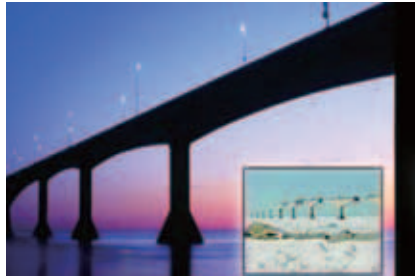
Canada- Prince Edward Island Confederation Bridge Below freezing temperature installation
