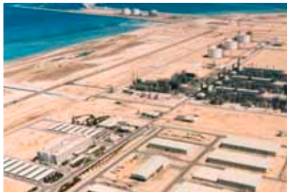
Qatar Las Raffan Gas plant Dowelling of foundations
