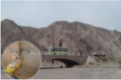
China- Gansu Bridge renovation and structural crack repair
