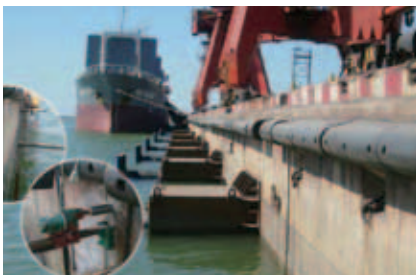
China- Liaoning Seaport Damp condition large diameter fender anchoring
