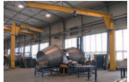
Germany Crane anchoring
