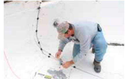
U.S.A.- California Active leak repair
