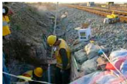
China- Shandong High speed railway line, Addition of electrical line poles
