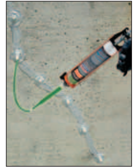
For Leaking Cracks
