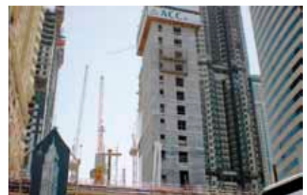
UAE- Dubai Elite Tower Dowelling of floors to core wall
