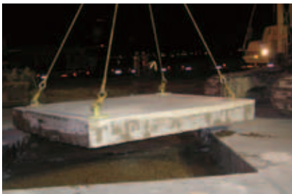
USA- California Oakland International Airport Lifting slabs in runway repair
