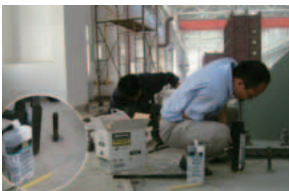
China- Tianjin Factory equipment anchoring
