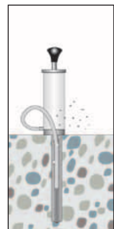
2 Clean hole with a blow pump.
