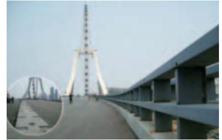
China- Tianjin Highway crash barrier anchoring
